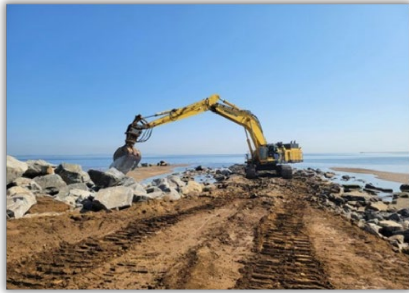
Union Beach, NJ Groin Construction
