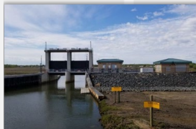
Port Monmouth, NJ Completed Tidal Gate
